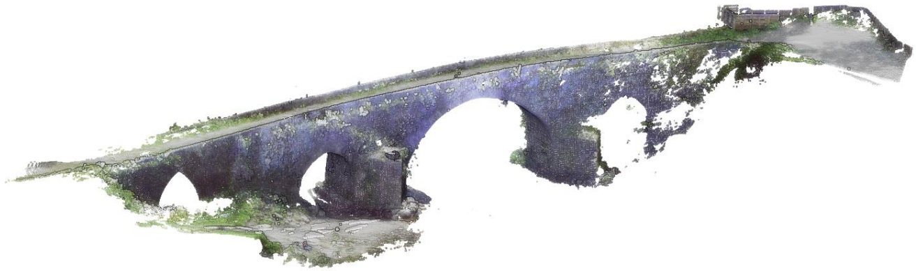
Fig. 4. Point cloud of the bridge cleared of surrounding vegetation and noise.
