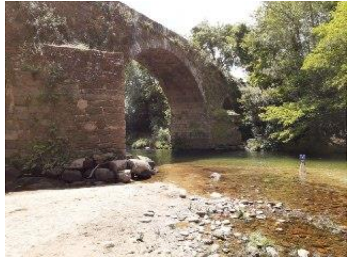
Fig. 1. Photograph of the north side of the bridge (May 2021).
